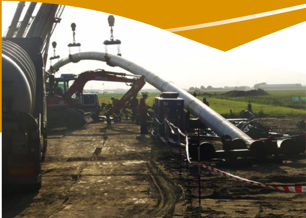
Start HDD-boring
